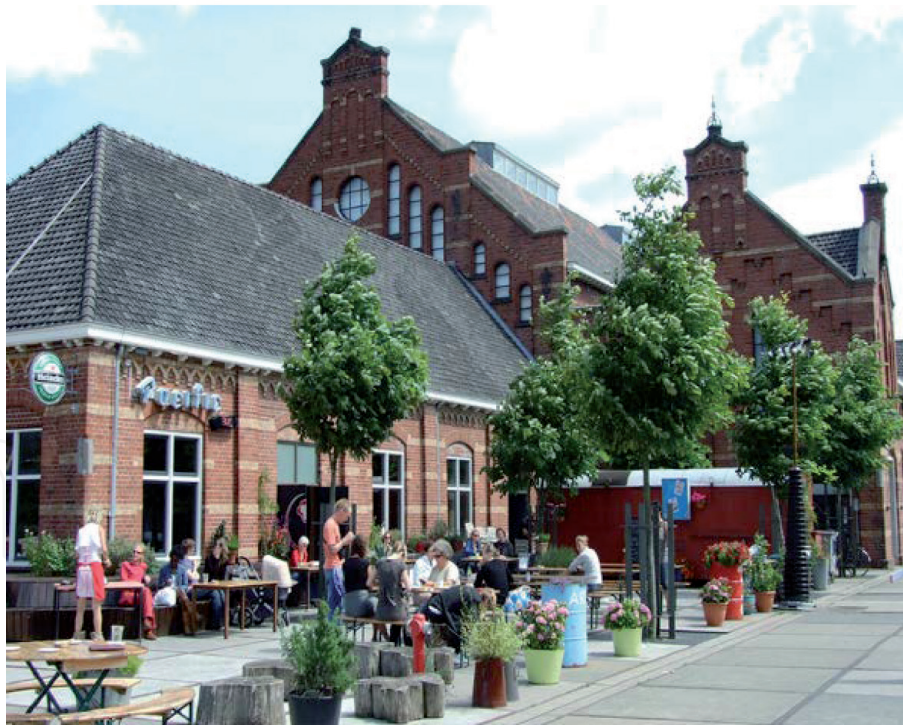
Figure 4. Westergasfabriek, Amsterdam, channel side view. Loures [21, 22].
