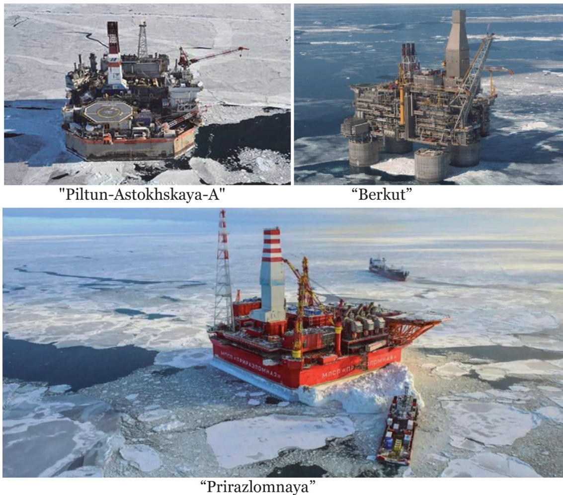
Figure 1. Large offshore platforms in Russia.
