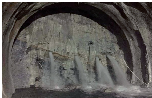
Figure 6. Water inrush in the tunnel after the advanced drilling.
