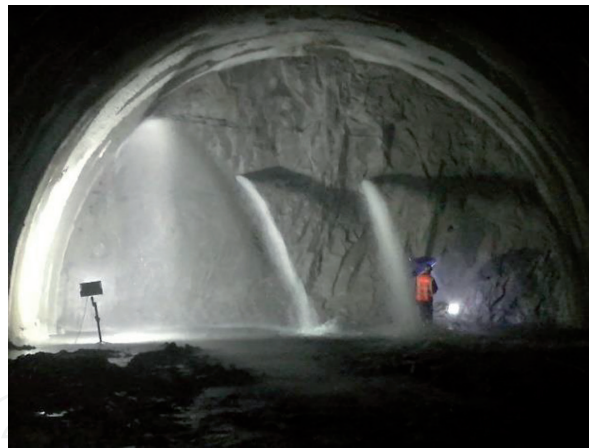
Figure 6. Water inrush in the tunnel after the advanced drilling.
