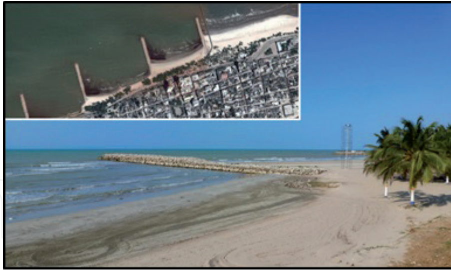
Figure 16. Example of sandy beach at Riohacha, accreted updrift by the help of jetties.
