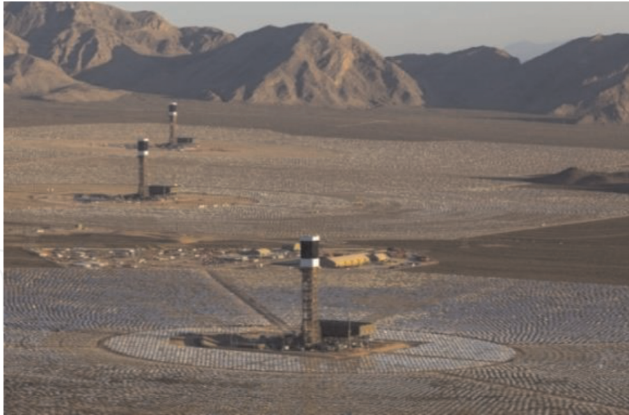
Figure 6. Ivanpah: the largest CSP plant in the world [16].
