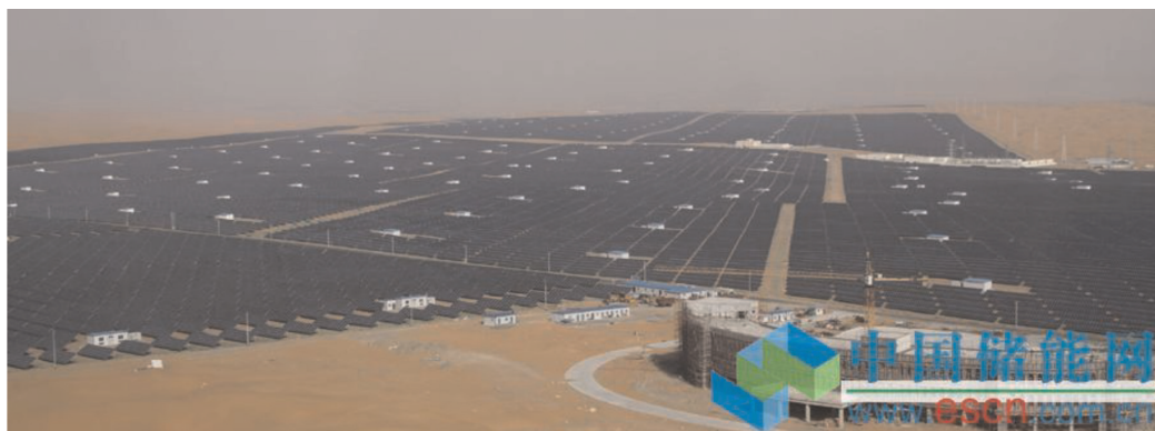
Figure 3. 1500 MW Tengger Desert solar power plant in China.
