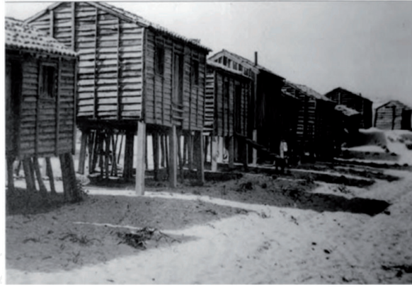
Figure 13. Flood-proof piling houses built on the coast of Tocha-Mira, Portugal, in the mid-nineteenth century (Adapted from [28]).
