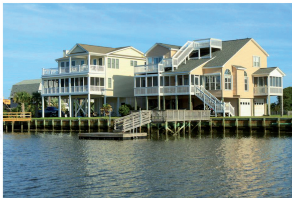
Figure 15. Two luxurious waterfront homes built on pilings over the water in the USA ( https://www.homestratosphere.com/houses-built-on-stilts/ ).
