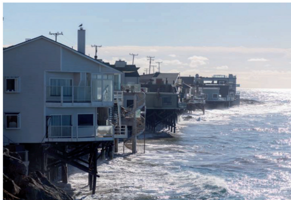
Figure 14. Houses on Malibu beach built on pilings with waves crashing underneath the houses ( https://www.homestratosphere.com/houses-built-on-stilts/ ).
