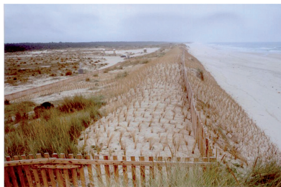
Figure 8. Rehabilitated stretch of the Leirosa sand dunes system, from May to September 2000 (Adapted from [12]).
