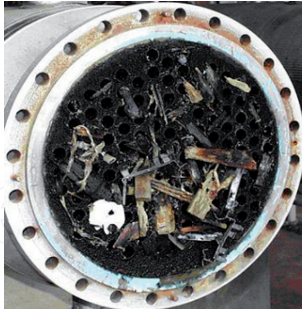
Figure 7. Accumulation of solid particles in the plate of a tubular heat exchanger (Source: By courtesy of AH&C Heat Transfer Solutions Inc.).
