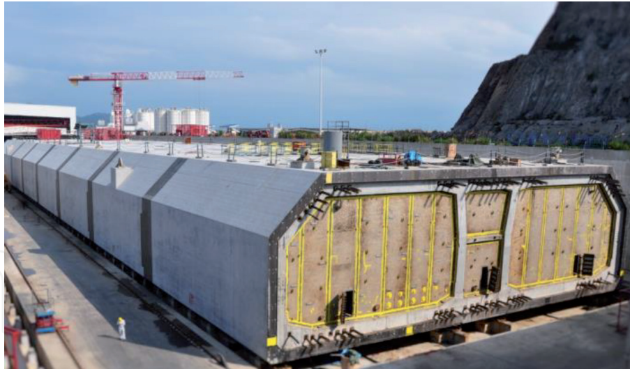
Figure 10. Photo of immersion joint of tunnel element in HZMB Island-tunnel project.
