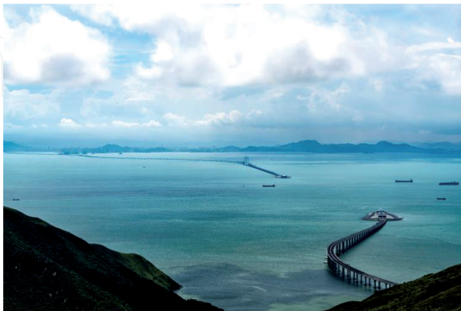
Figure 1. Overview of HZMB link from Hong Kong side.
