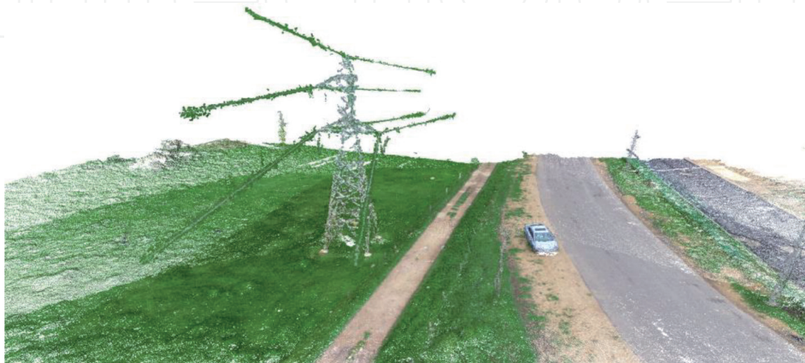
Figure 15. Results of 3D reconstruction of electrical infrastructure.
