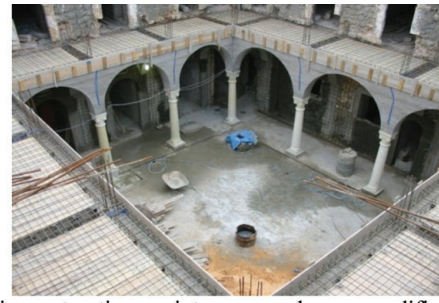
During restoration, maintenance and space modifications
