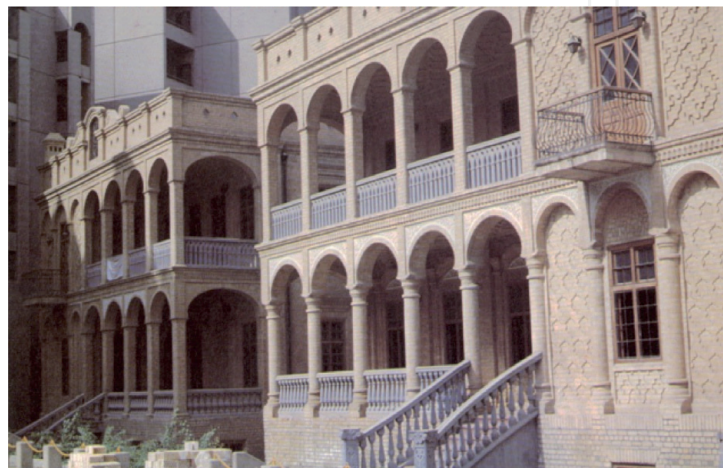
Figure 6. Traditional Baghdadi houses that have been rehabilitated for administrative use.
