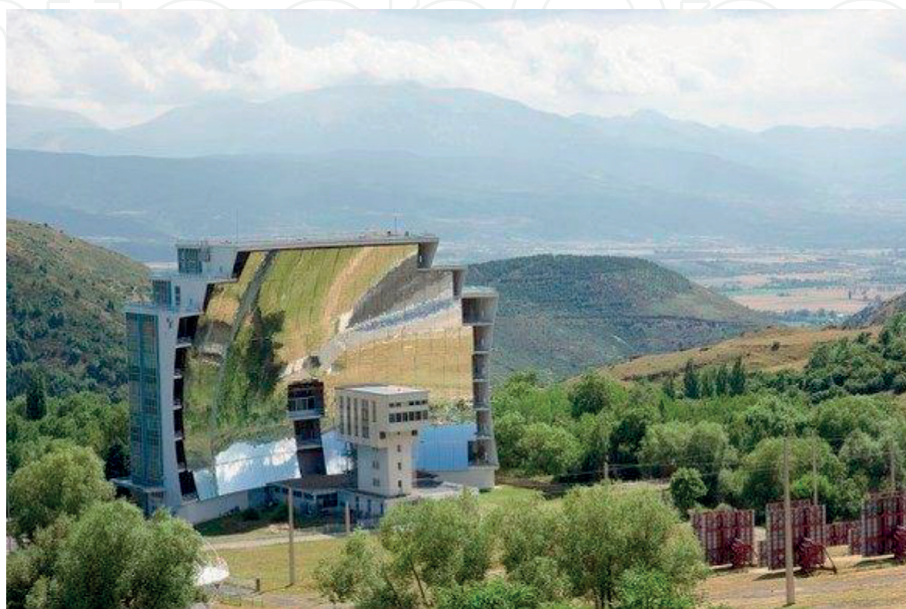
Figure 1. General view of the France furnace.
