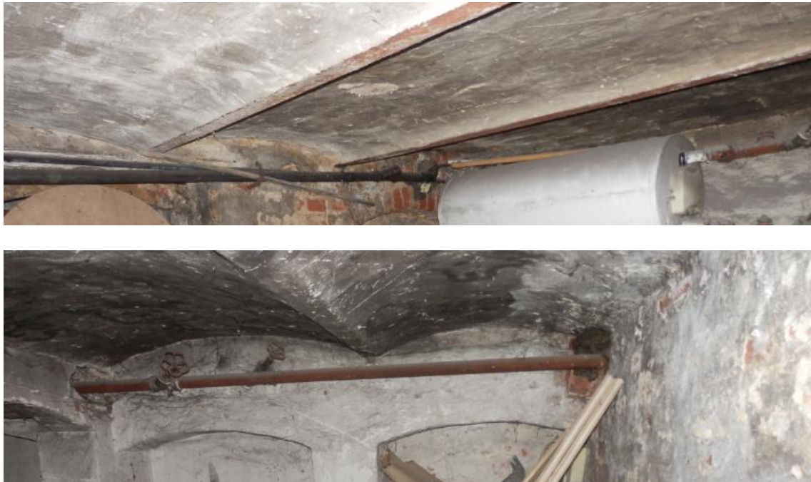
Figure 4.53 Floor above the basement.
