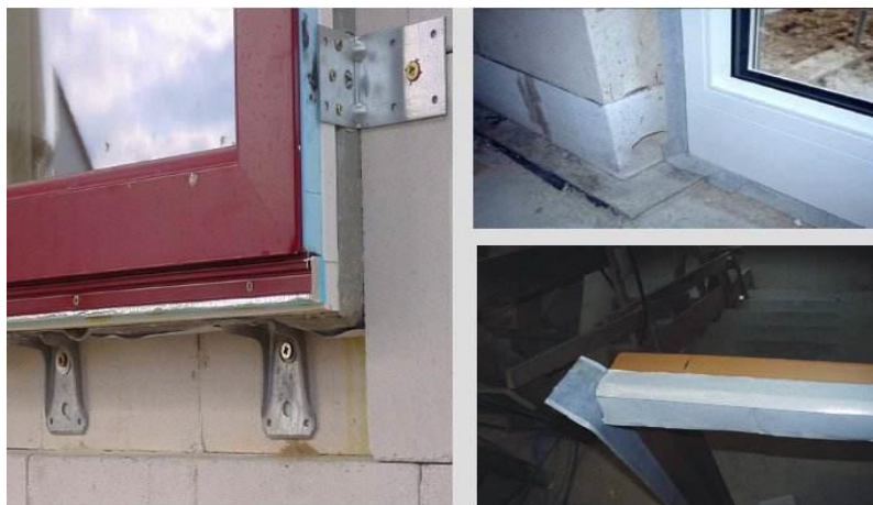
Figure 2.16 Mounting angle iron (on the left) and sealing tape (on the right)
