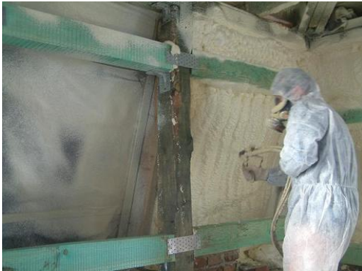
Figure 4.48 Spraying of polyurethane foam between the structural elements of the roof
