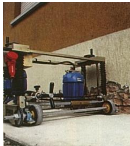
Figure 4.61 Propellered Platform electric saw used to walls undercut
