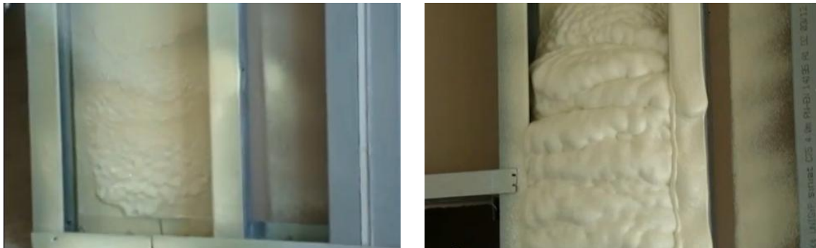
Figure 4.30-31 Filling the space between profiles by polyurethane foam.
