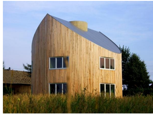
Figure 2.2 Design of houses in the village Pszczyna shape of the house cube. (Poland, Silesia, project of Robert Konieczny) Source: http://projektowaniewnetrz.eu/akademia2/wp-content/uploads/2012/04/indywidualny-dom-typowy-1.jpg
