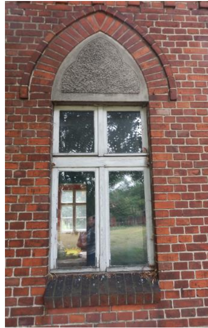
Figure 4.41 Lintels in considered building Source: Own
