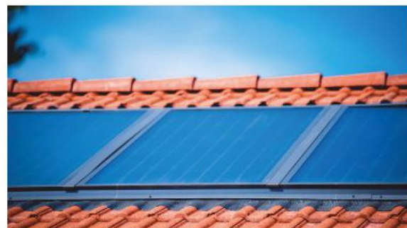
Figure 4.82 Flat roof collector in the fitting.
