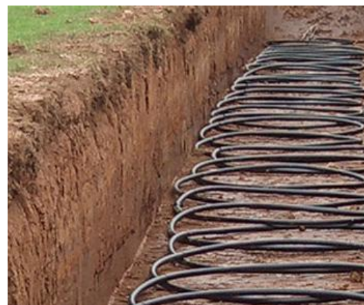
Figure 3.10 Ground Source Heating Pipes Source: http://www.simonlawrencebuilders.co.uk
