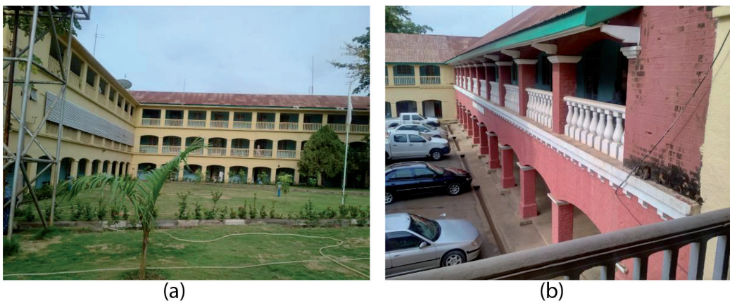
Figure 7. (a) Kaduna state Ministry of Health and Human Resource building and (b) Kaduna State Ministry of Women Affairs building at the foreground.
