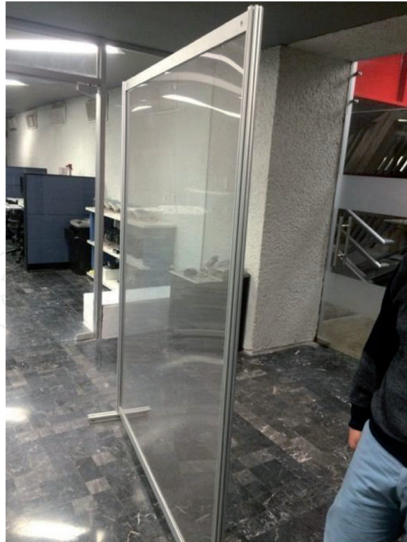
Figure 5. Transparent acrylic mounted on an aluminum base.
