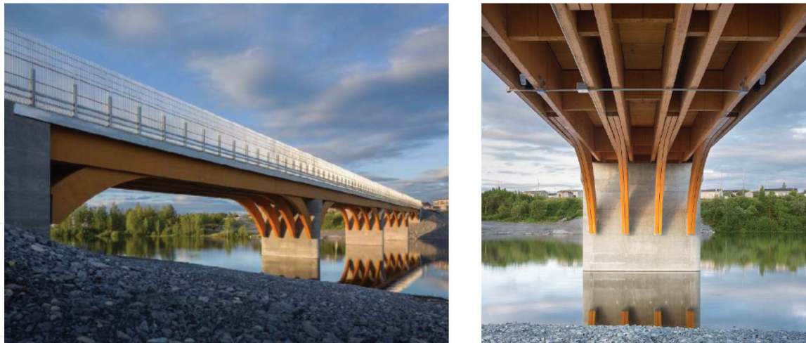
Figure 8. 160-m-long timber bridge with GLT deck structure in Mistissini, Canada. (Source: Photos obtained from Lefebvre and Richard [13]).
