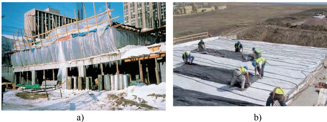
Figure 1. (a) Concrete in cold weather. (b) Cold weather curing.
