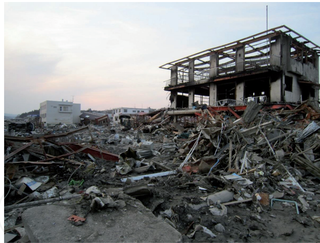
Figure 1. Damages by 2011 East Japan earthquake (after associate professor Sakamoto of Nagoya University).
