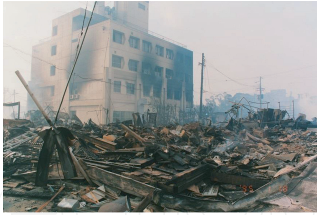
Figure 7. Collapses of buildings in Kobe at 1995 Kobe earthquake (after Kobe damage database).
