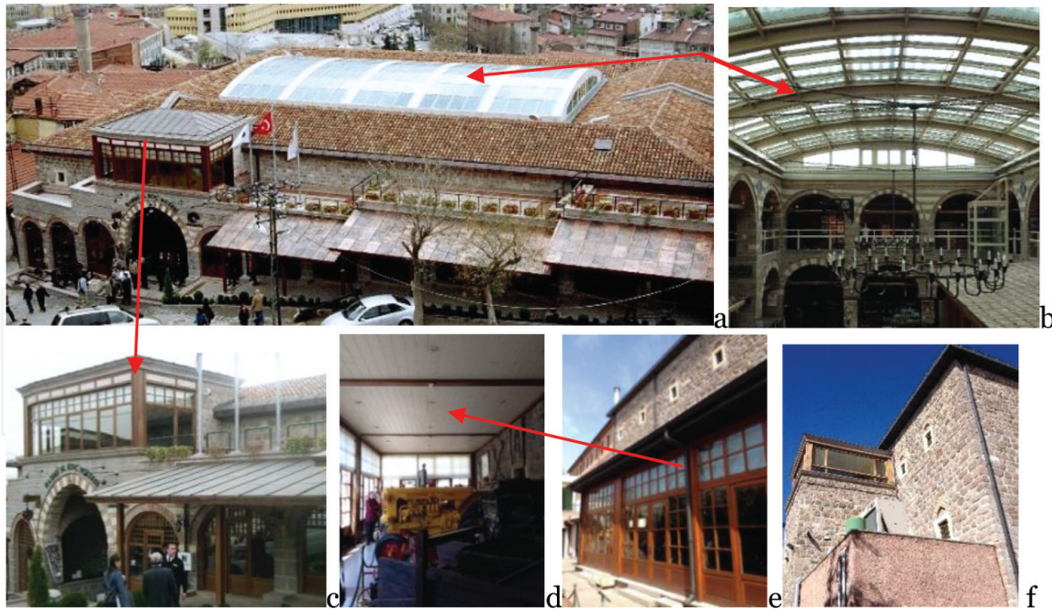
Figure 5. Çengel khan: Rooftop addition covering the courtyard, exterior (a) [56] and interior views (b), completion of side walls above the entrance vault and storefront additions (c) and views from rear additions (d, e, and f) [39].
