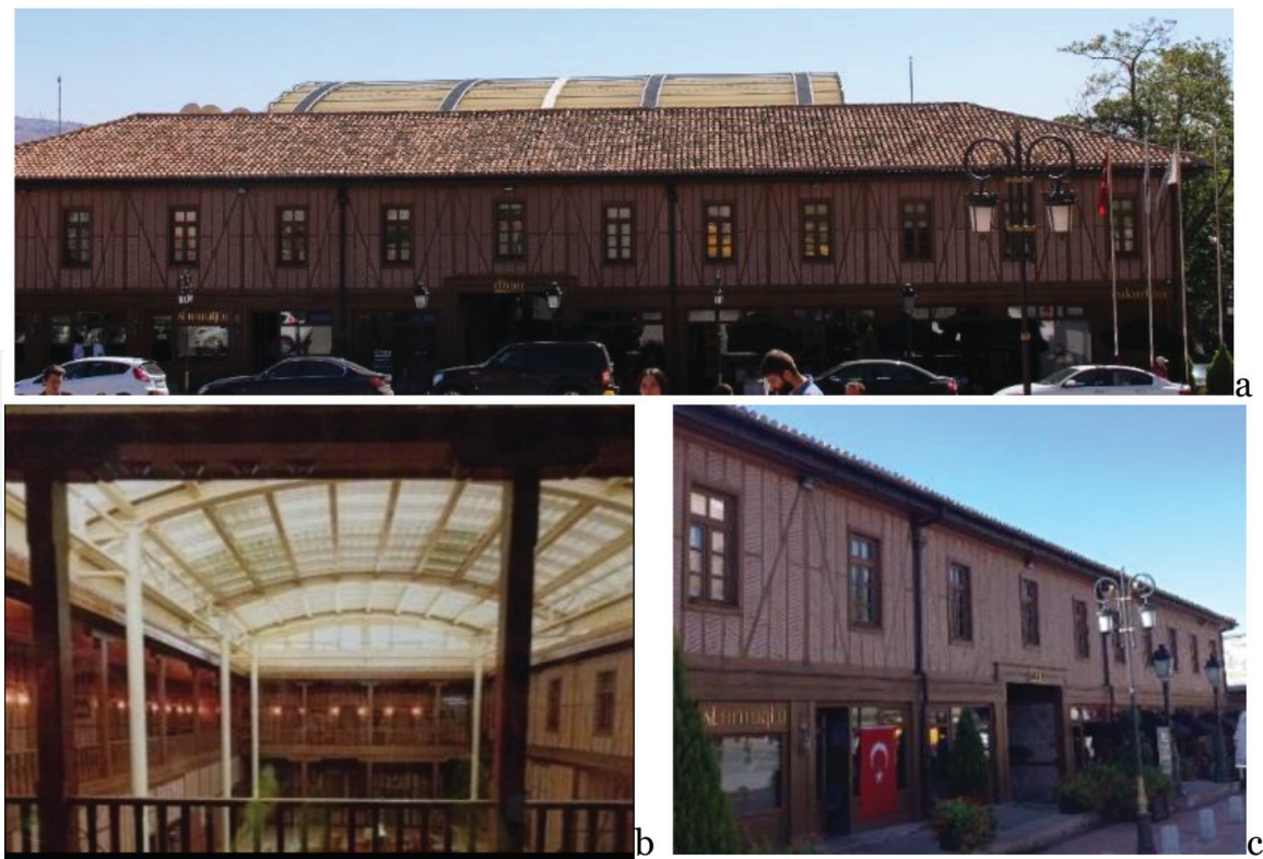
Figure 12. Çukur khan: Rooftop addition (a and b) and storefronts (c) [39, 57].
