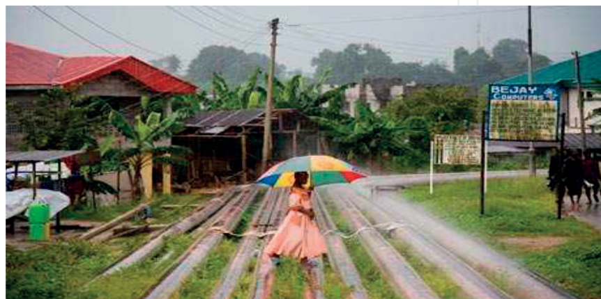
Figure 4. Oil pipelines in Okrika community, Niger Delta [55].
