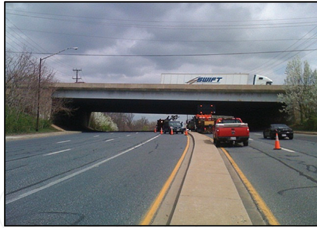
Figure 3. Maryland bridge carrying I-270 over Middlebrook Road.
