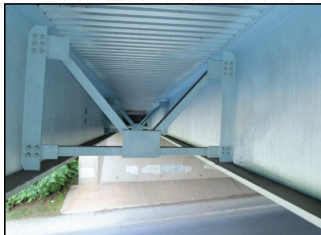
Figure 4. K-type cross brace on Middlebrook Bridge.
