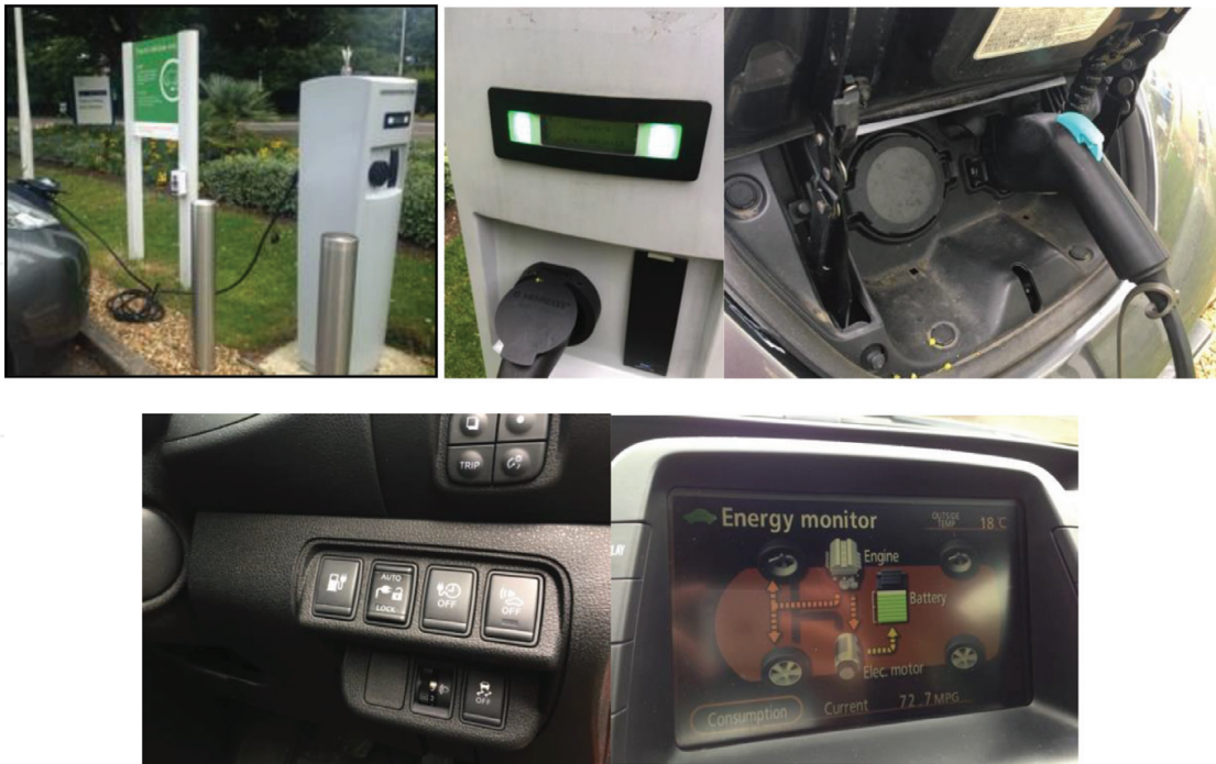
Figure 6. (a)–(e). On-site WPC facilities and charging compatibility.
