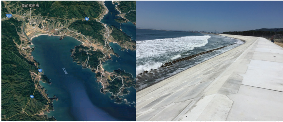
Figure 10. Current situation of defense construction along the Tsunami-hit coast.
