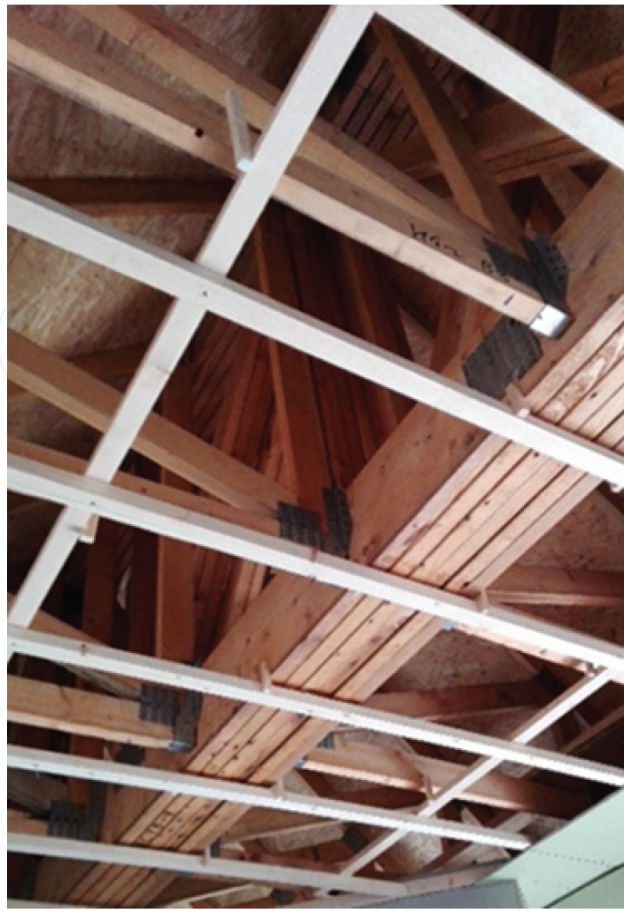
Figure 1. Application of girder truss in building structure.
