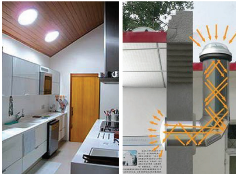
Figure 9. Solar light pipes system. Source: Google Search—Images.
