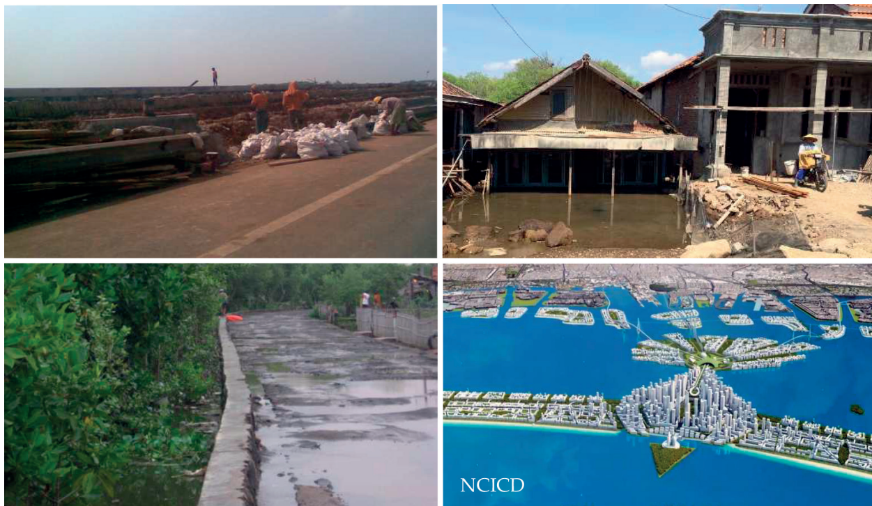
Figure 8. Short- and long-term mitigation and adaptation against the consequences of land subsidence (e.g. elevating roads and housing, and building dykes, mangrove areas, and giant sea walls) (sources: authors, [12, 16]).
