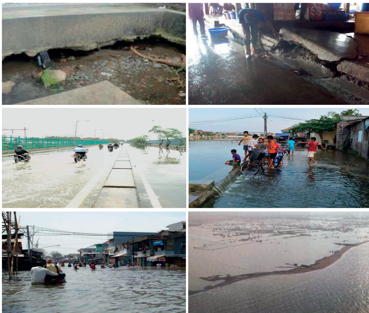
Figure 3. Example of documentation of the impact of subsidence such as cracks in buildings and infrastructures, and tidal inundation (sources: [12, 13]).
