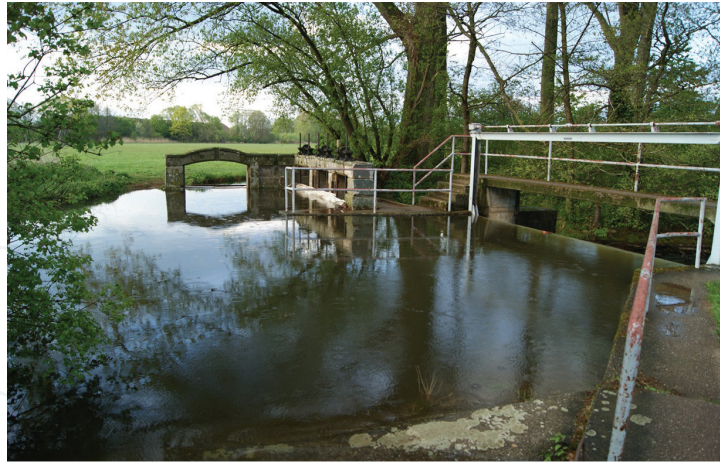
Figure 2. Main sluice (near Mörlheim) along the river Queich (right side of the photo). The sluice is closed which allows water to flow into a main ditch (upper left side of the photo; photo: Martin Alt).
