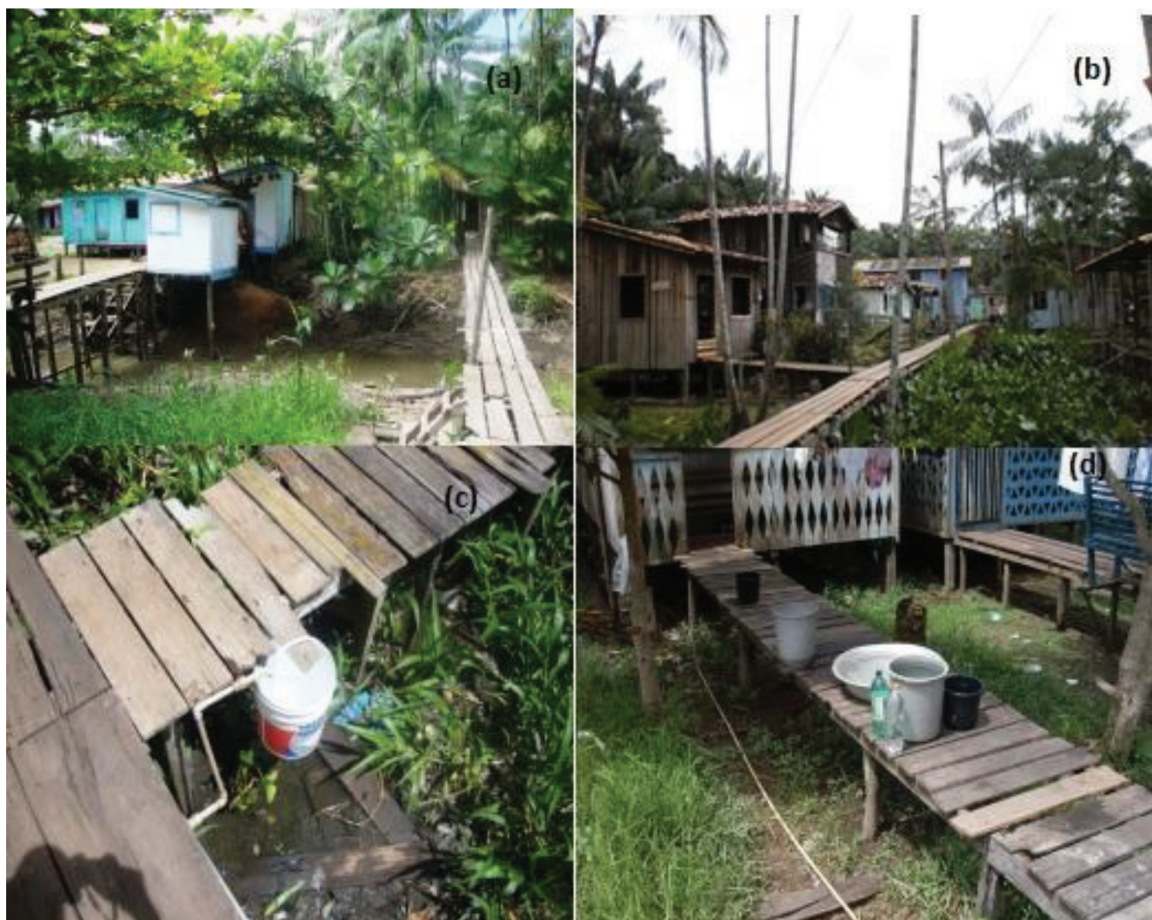
Figure 3. Urban area that represents an environmental and sanitary risk to the residents. (a) Stilt houses and precarious wooden bridge to access the houses, (b) residence with wooden bridge, (c) and (d) precarious access to water and environmental and health vulnerability. Source: collection of the Laboratory for Studies of Cities—UNIVAP [10].
