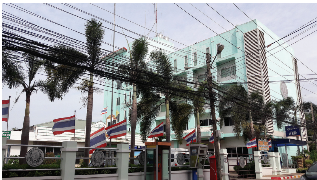
Figure 7. Kho-hong municipality office.
