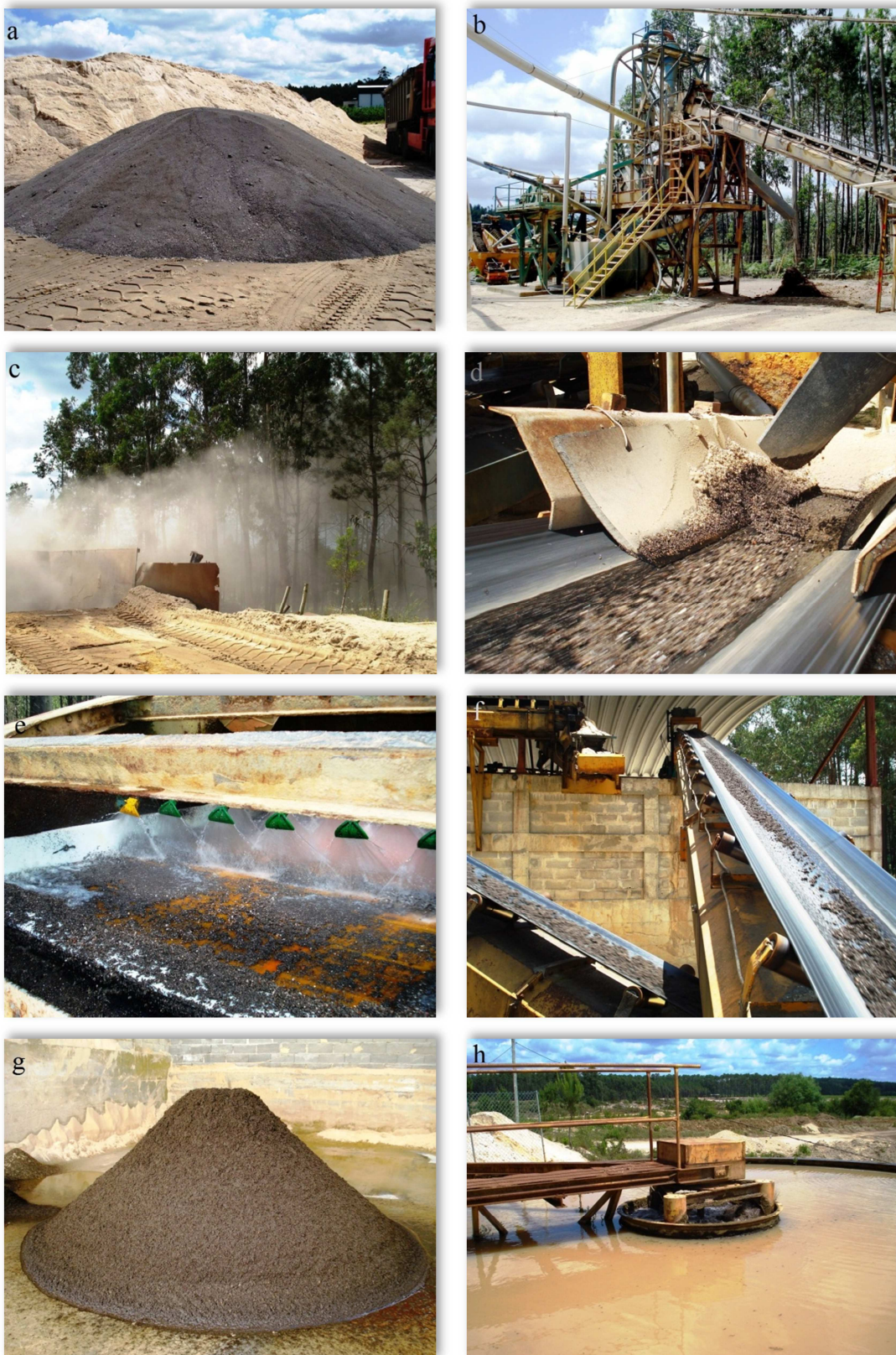
Figure 2. 3. Industrial test for bottom ash treatment. (a) Raw bottom ash (BA) storage, (b) Washing and sieving installation, (c) Initial stage of the treatment and dust generated during introduction of bottom ash in the treatment process, (d) Bottom ash processing, (e) Bottom ash washing stage; (f) Conveyor belts and sieves that make the separation of bottom ash particles by size fractions; (g) Useful particle size ( < 1000 \mu\text{m} ) after bottom ash treatment, (h) Washing liquid effluent treatment by sedimentation.
