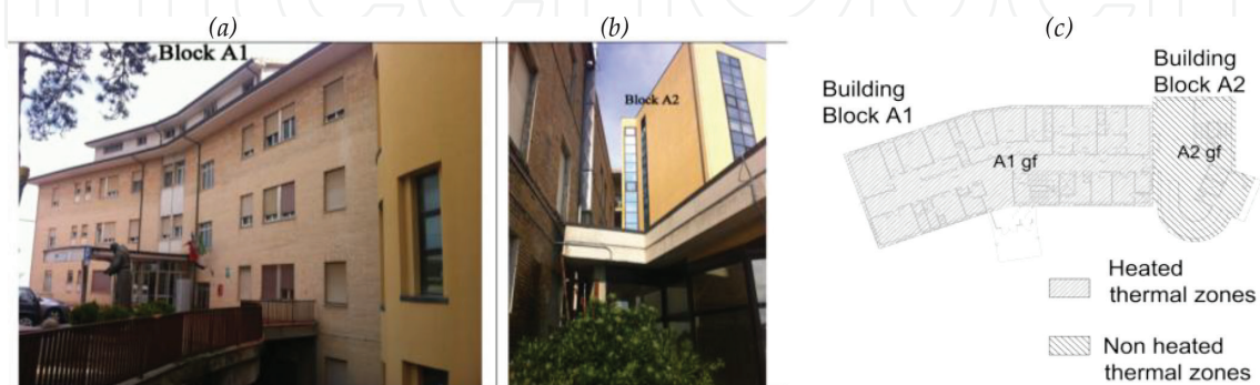
Figure 1. Front view of block A1—Partially hidden by block A2 (a), rear view of block A2 at the point where it connects with block A1 (b), and plan of the ground floor (c).
