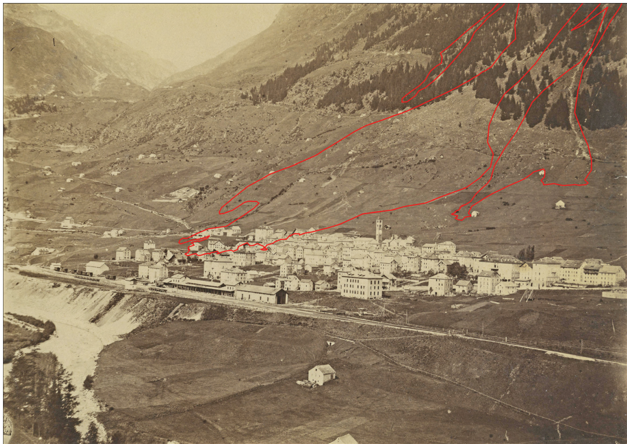
Figure 4. The Sasso Rosso slope failure (Airolo, 1898). Projection of the slide perimeter on an oblique terrestrial image of the area prior to the event (source: Conedera et al. [21]).
