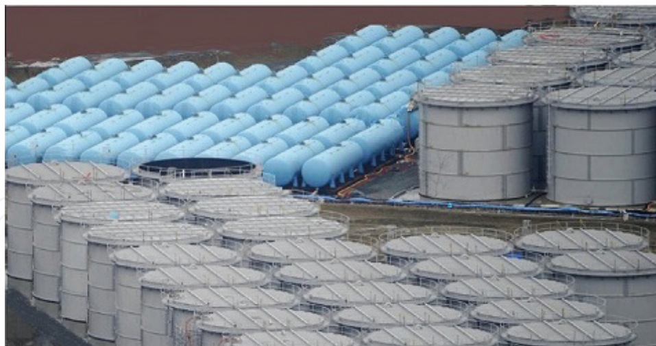
Figure 4. Fraction of tanks with >300,000 m 3 contaminated water at Fukushima power plant.
