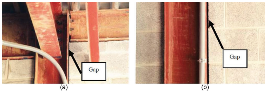
Figure 3. Example of partition infill wall isolated from the frame with small gaps: (a) beam-column joint area and (b) gap between column and infill wall [Photo by Ali M. Memari].
