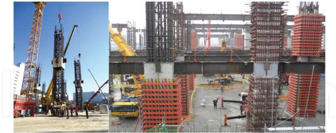
Figure 2. Semiconductor FAB (weld-connected PSRC composite column).
