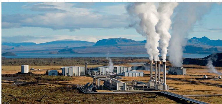
Figure 1. Geothermal energy plant [12].
