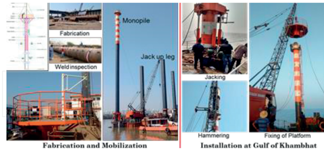
Figure 5. Installed LiDAR at Gulf of Khambhat for MNRE-NIWE.
