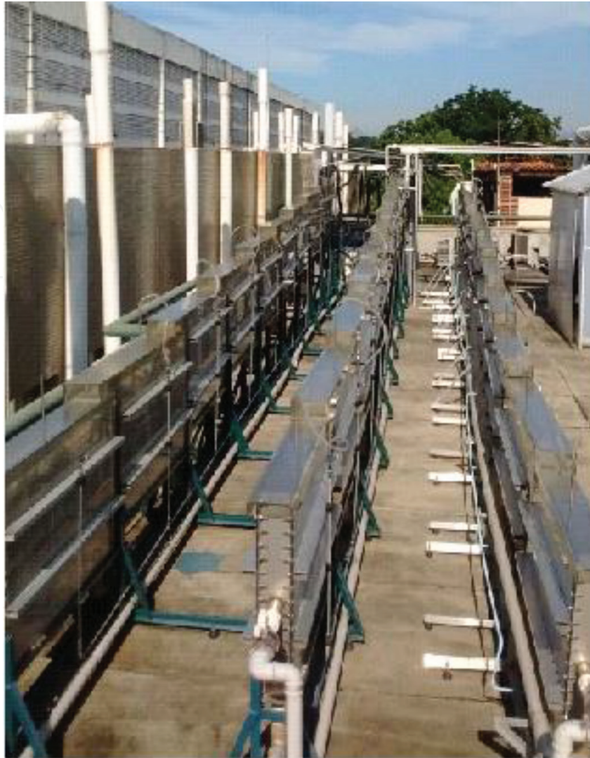
Figure 5. Photobioreactors at GreenTech.
