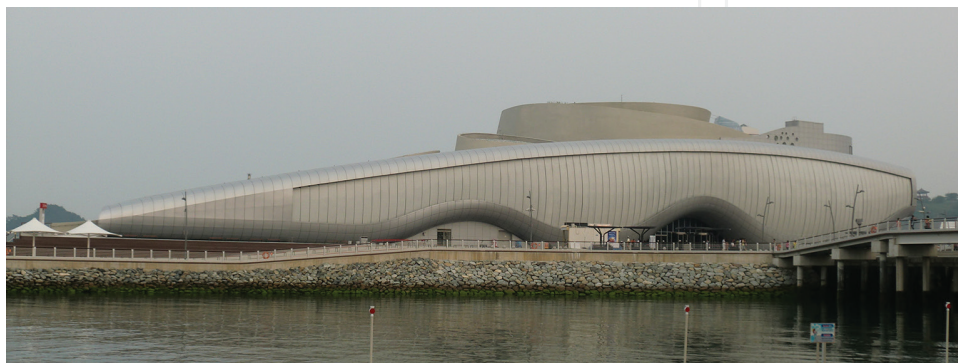
Figure 13. The kinetic façade and closed lamellas [47].
