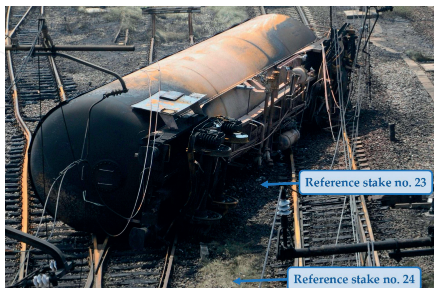
Figure 13. Rear view of carriage no. 1 in the accident scene and positions of track reference stake nos. 23 and 24.
