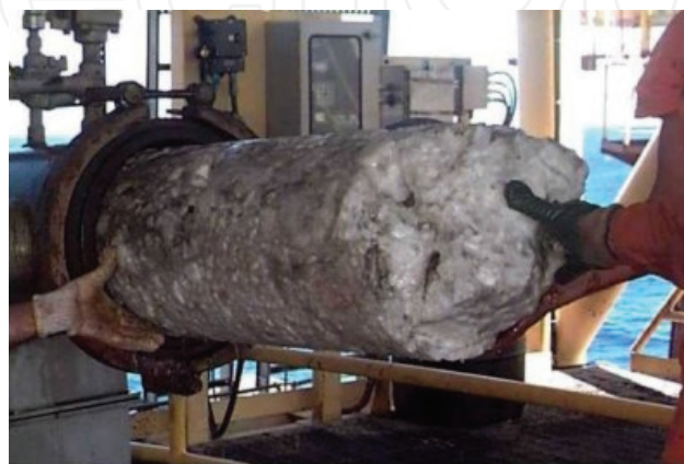
Figure 1. Recovered gas hydrate plug from a subsea pipeline off the coast of Brazil (courtesy of Petrobras).
