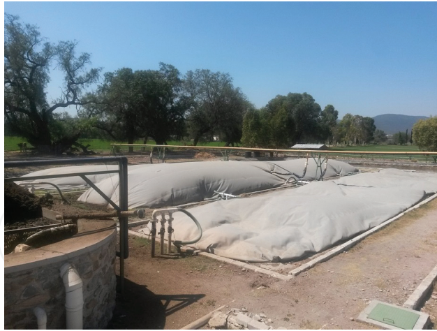
Figure 2. Covered lagoon digesters for cow manure treatment.
