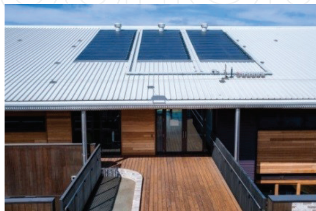
Figure 2. Air-based PVT collectors implemented in a net-zero energy office building.
