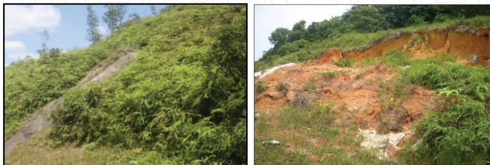
Figure 1. Condition and appearance of stable and unstable slopes soil.
