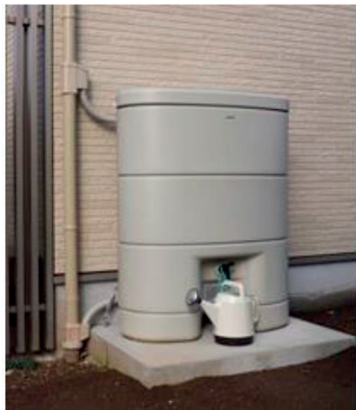
200-liter rainwater tank
