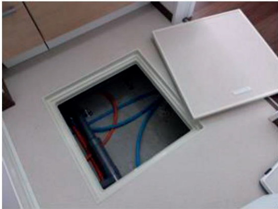
Underfloor inspection opening
