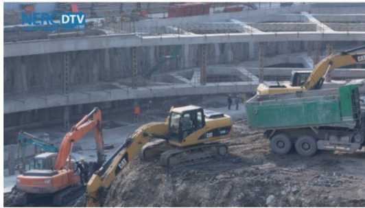
c) Construction Field
