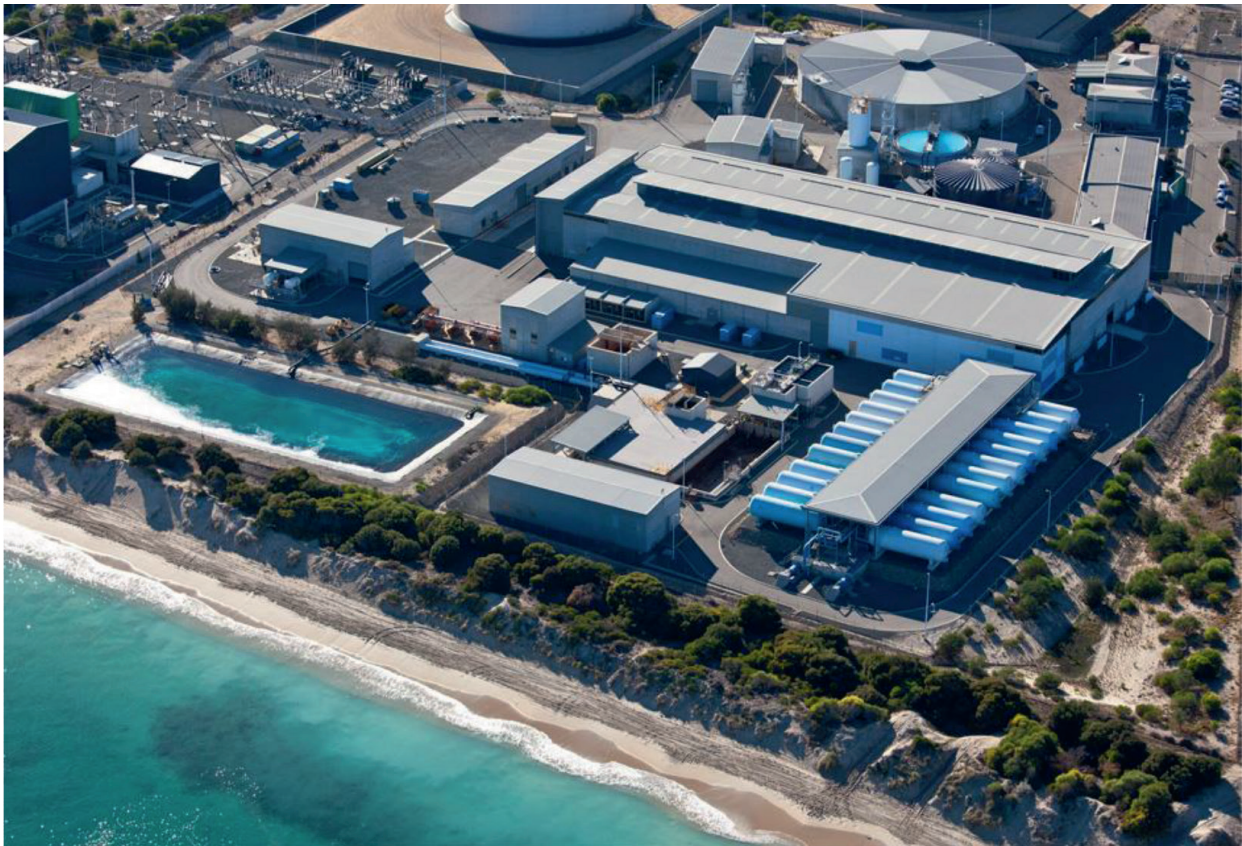
Figure 5. Perth desalination plant.
