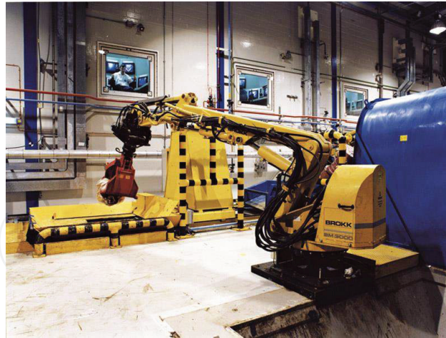
Figure 1. A BROKK robot, equipped with a gripper, being used for a pick and place task at the Sellafield nuclear site in UK. Human operator can be seen controlling the robot from behind a 1.6m thick lead-glass window which shields him from radiation, but significantly limits his situational awareness. For more examples, refer to www.sellafieldsites.com/solution/decommissioning .
