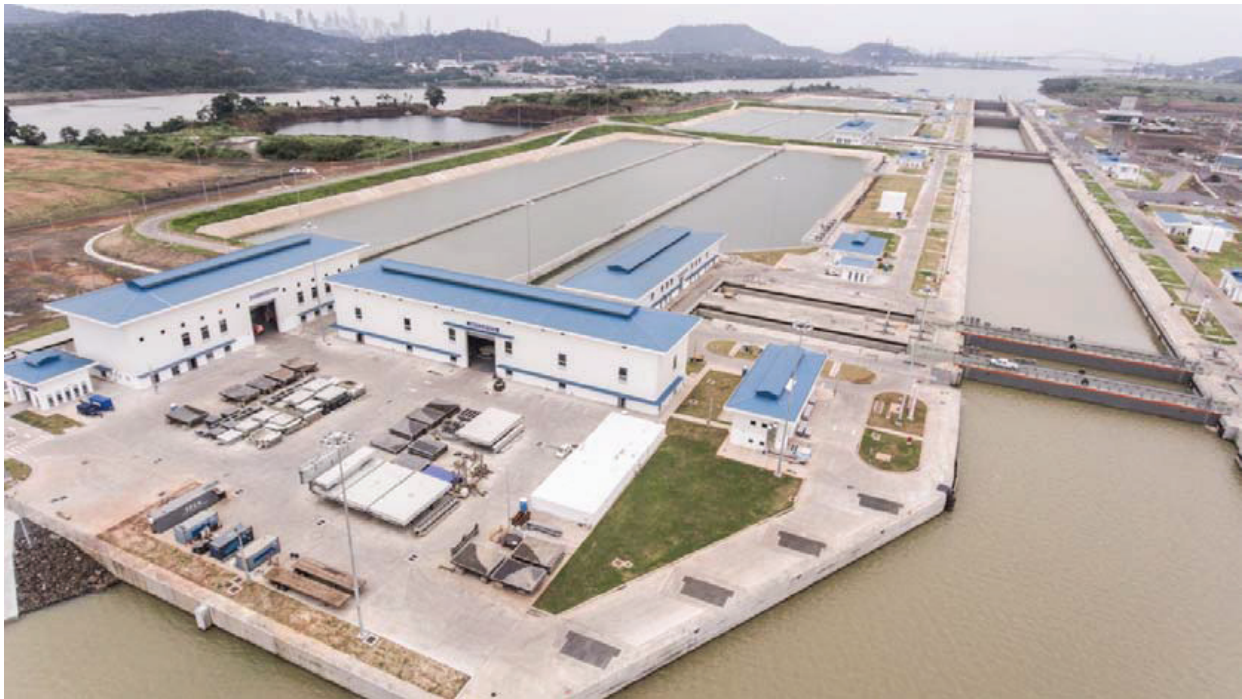
Figure 10. Overview of the structure where the two gates are located at each end of the chamber.
