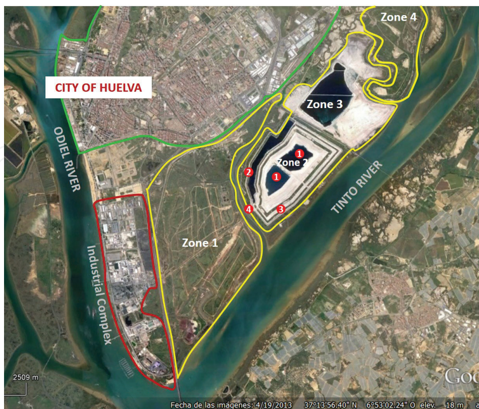
Figure 2. Aerial photograph of the area of the Tinto river marshes. (1) Settling ponds, dumping area of FY; (2) regulating reservoir, (3) perimeter channel, and (4) pumping station.
