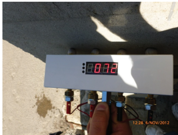
Figure 9. The measurement of a concrete pillar, second measurement.
